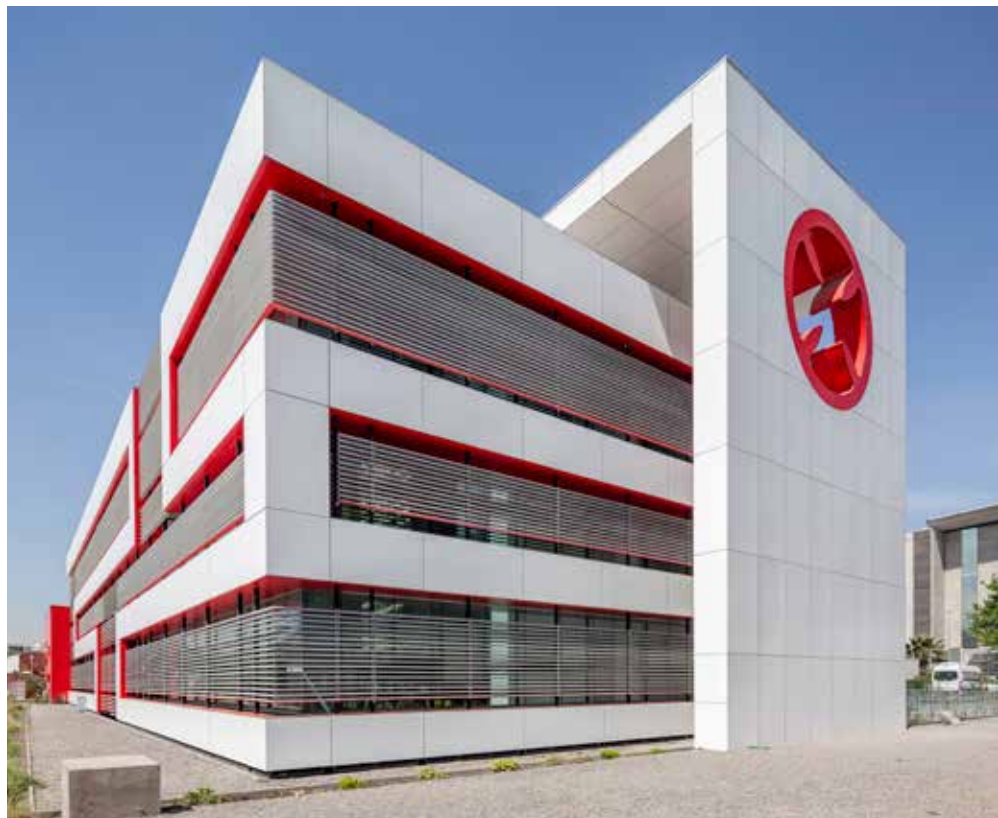
THE FAÇADE OF THE TELETÓN HEADQUARTERS IN SANTIAGO IS CLAD WITH THE FOUNDATION'S COLOURS
