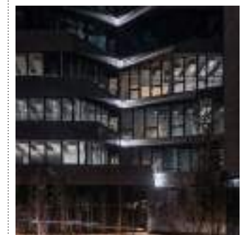
Details of the Nishi (top) and Higashi buildings (bottom)
