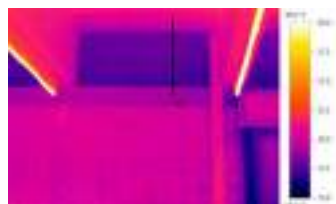
ORIGINAL NON RENOVATED BUILDING Interior wall surfaces are cold. Performance varies greatly, with significant energy loss from the interior to the exterior.
