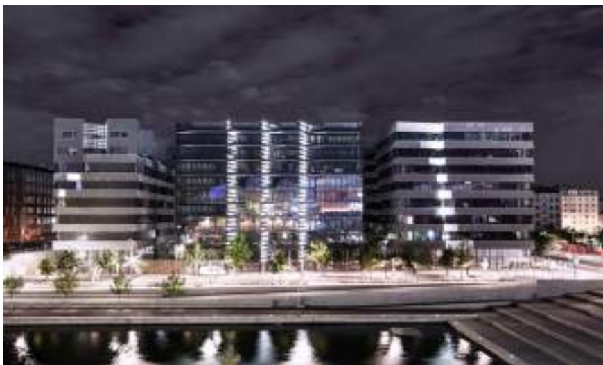
The Hikari buildings, from left to right: Nishi (Japanese for “West”), Minami (“South”) and Higashi (“East”)
