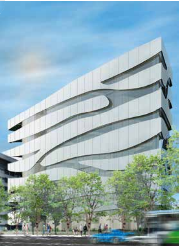
Working with AOA, Trespa designed an innovative façade solution for a project called White Vitacura. The building mixes glass and Trespa® panels to create an energy-conscious, low-budget exterior.
