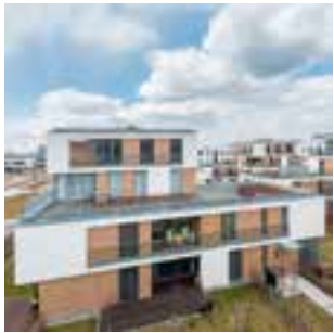
A mixture of concrete and Trespa® Meteon® Wood Decor panels animate the exterior of this residential complex, which exhibits a sharp form through its linearity.
