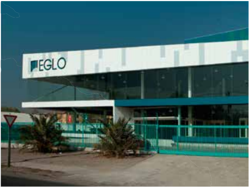
An earthquake in Chile in 2011 provoked the need to remodel Austrian company EGLO’s showroom and offices. Needing to reconstruct the building in a short amount of time without compromising quality, a mixture of colours and sizes of Trespa® façade panels were chosen to compliment the glass components in the new design.
