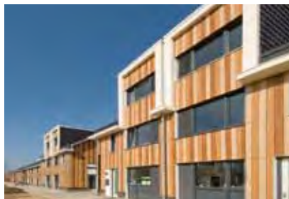
Building the largest Passive House development in the Netherlands
