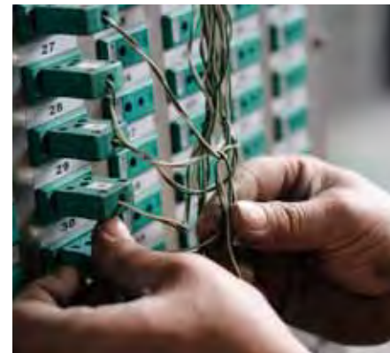
Probes connecting the measuring equipment
