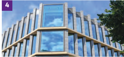
68-86 Farringdon Road – Offices
