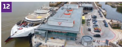
12 Isle of Man Ferry Terminal
