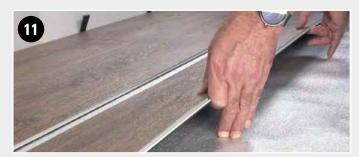
DISASSEMBLING LONG SIDE Wish to disassemble? Lift up the entire row, in the same angle as you did during installation, then slide apart the rows.
