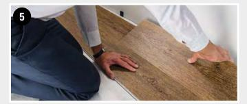
ENGAGE THIRD PLANK ON LONG SIDE Take another long plank (3). Repeating the previous step, insert the long side of plank 3 into the long side of plank 2. Then slide plank 3 to your left until the short side is in contact with the short side of plank 1.
