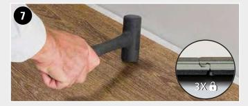
ENGAGE THIRD PLANK ON SHORT SIDE - 2 Using a soft-faced hammer slightly tap the joints on the short side to secure. This ensures 3x locking.
