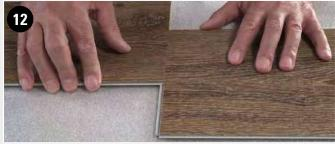
DISASSEMBLING SHORT SIDE Disassemble the row by sliding apart the planks on the short side.
