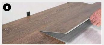
INSTALLATION FROM FOURTH PLANK ONWARDS For the next rows, installation does not require alternating rows. Install one row after the other by starting with angling the long side, until the short sides are in contact.
