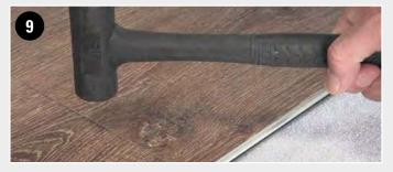
SECURING PLANKS As you go, don't forget to use a soft-faced hammer on the short sides to secure the locking.
