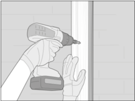
If the wall is flat and if no insulation is needed, then horizontal battens are not needed either (see next step).
