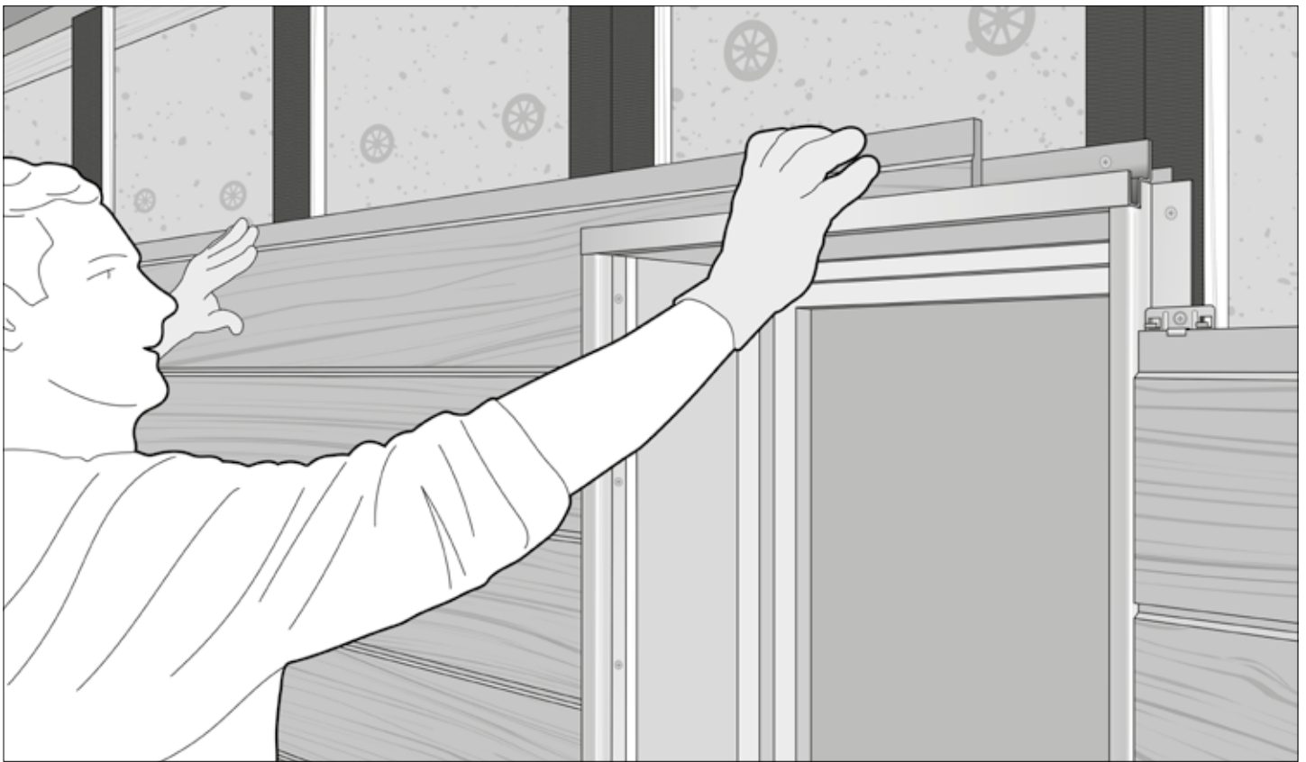
Work your way up next to the window. When you reach the top strip, trace the outline of the top of the window on to the back of the strip, and cut it with the jigsaw. Make sure the strip at the top of window lines up with the other strips in the row course and then secure with a clip.
