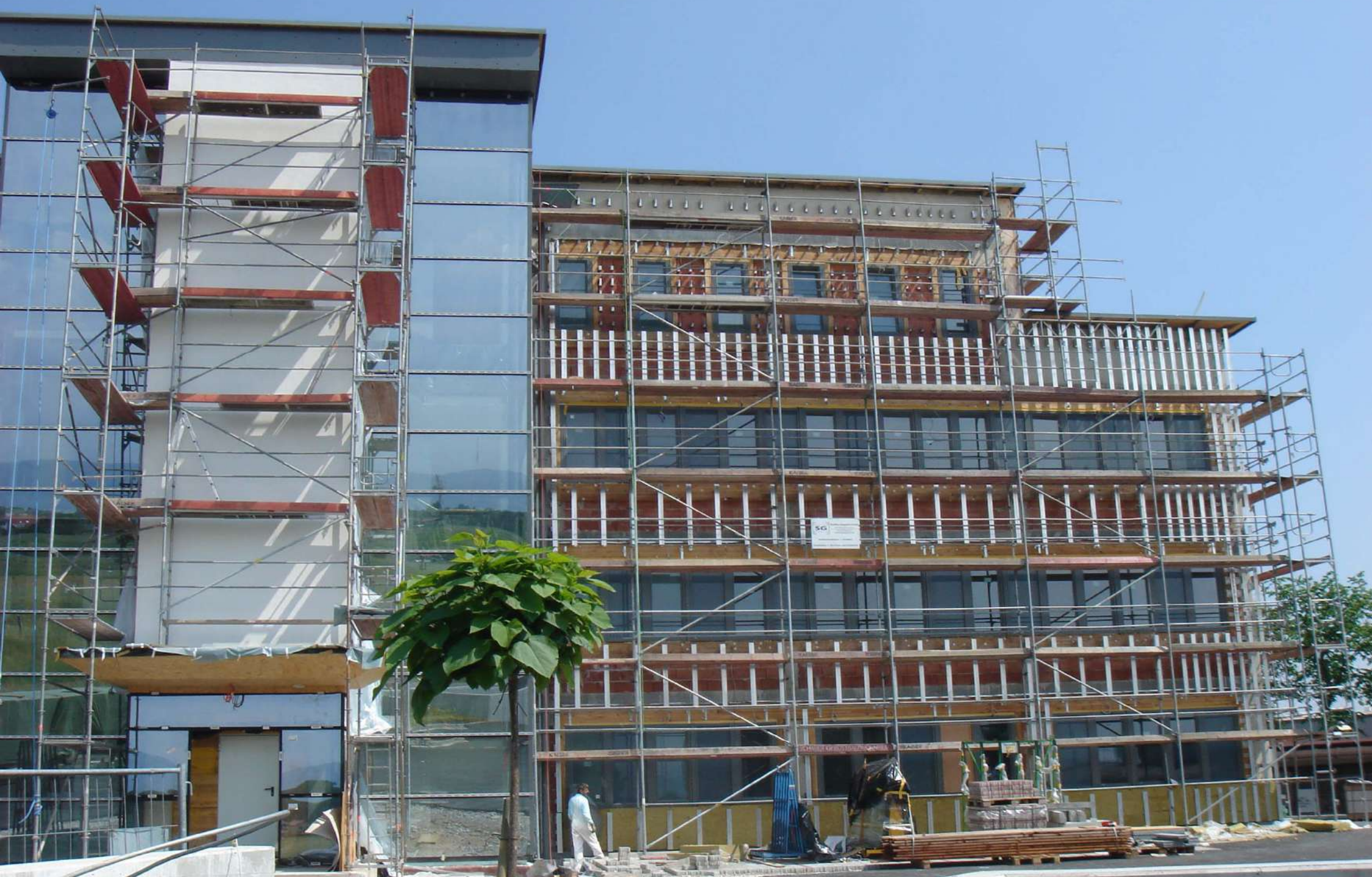
Office Building, Raaba / Austria, 1500 m 2 STO Ventec, F1.10
