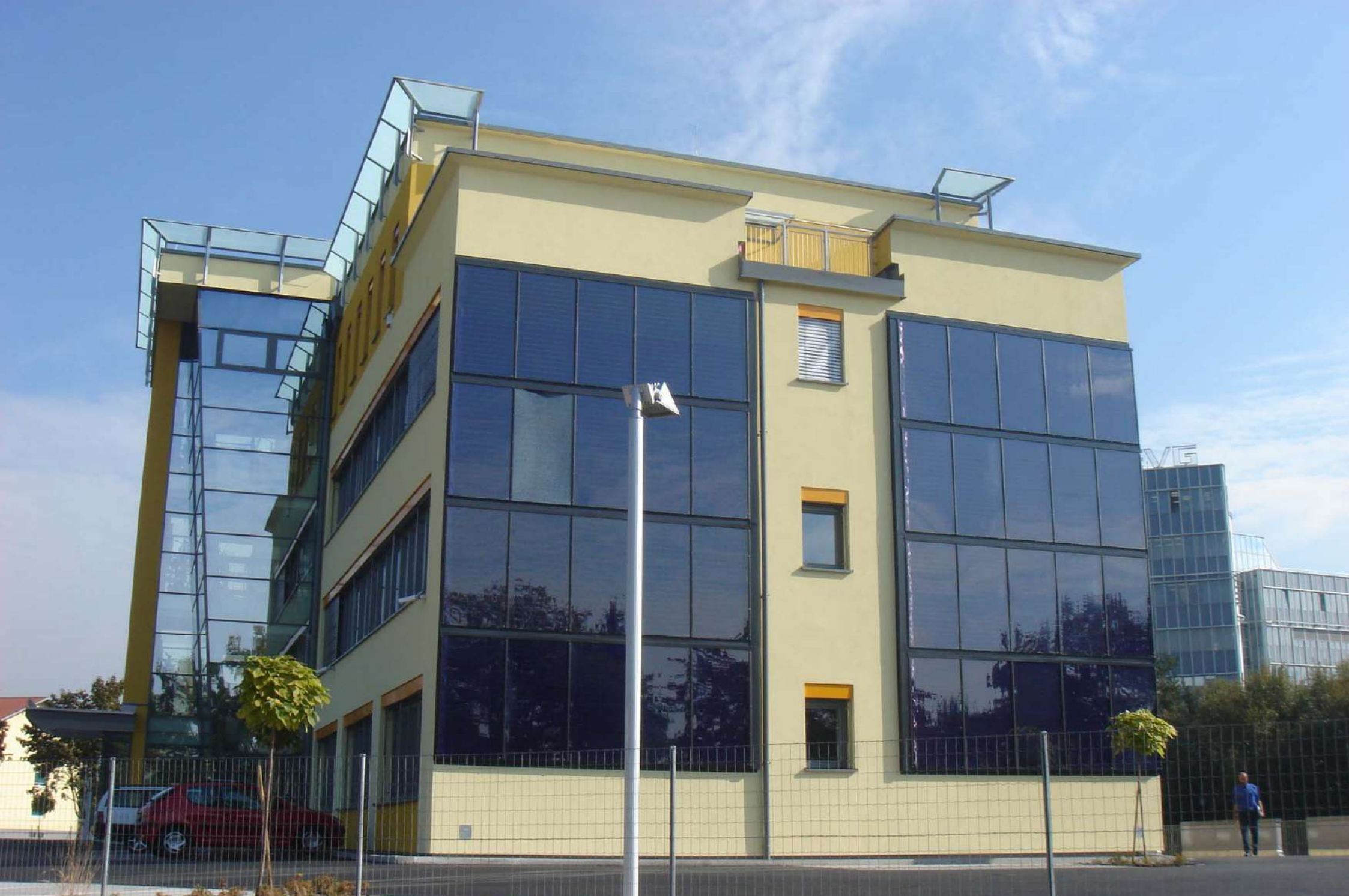
Office Building, Raaba / Austria, 1500 m 2 STO Ventec, F1.10
