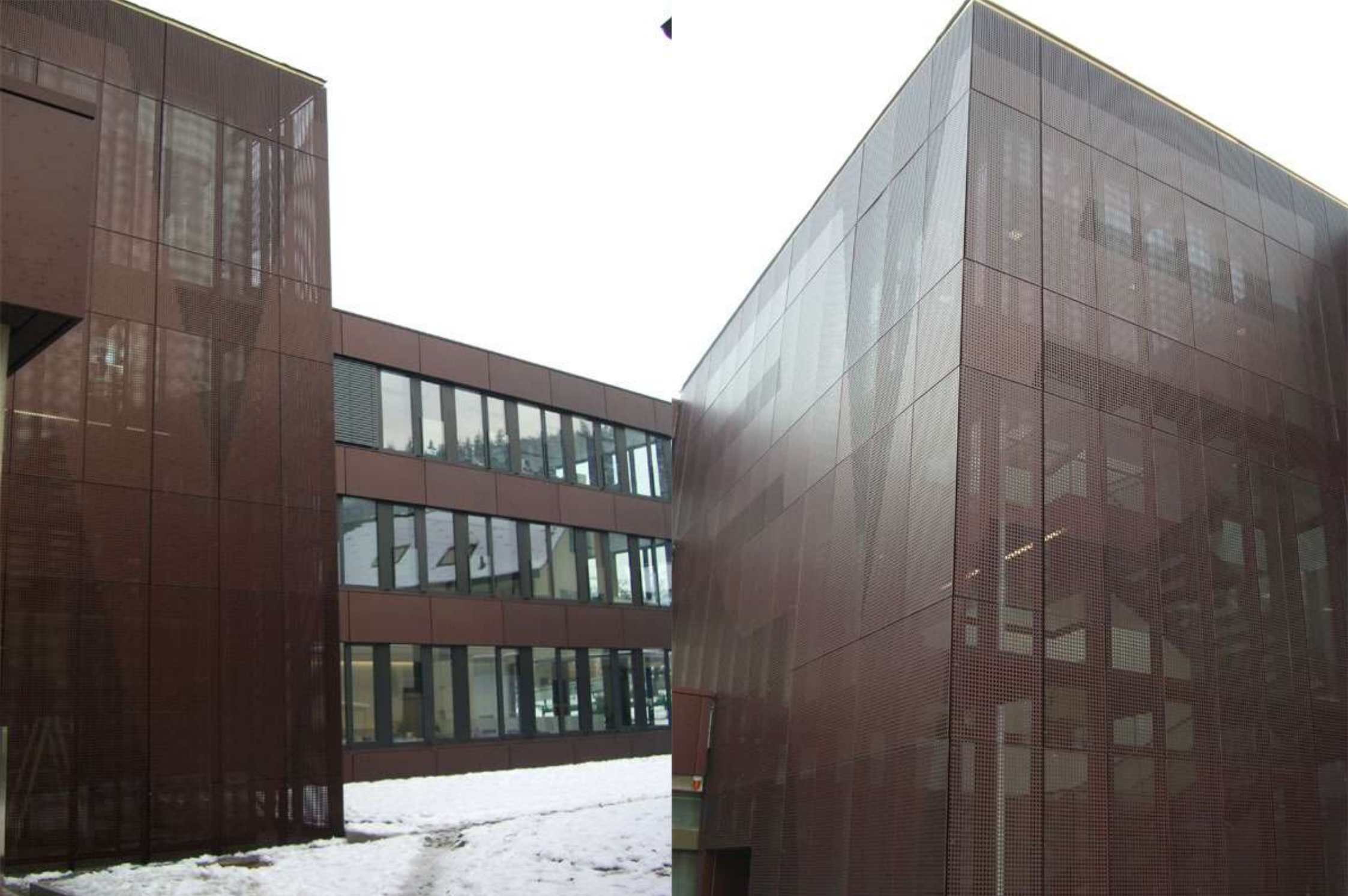
Bank, Rankweil – Austria, 1500 m 2 perforated Metal sheets, F1.10
