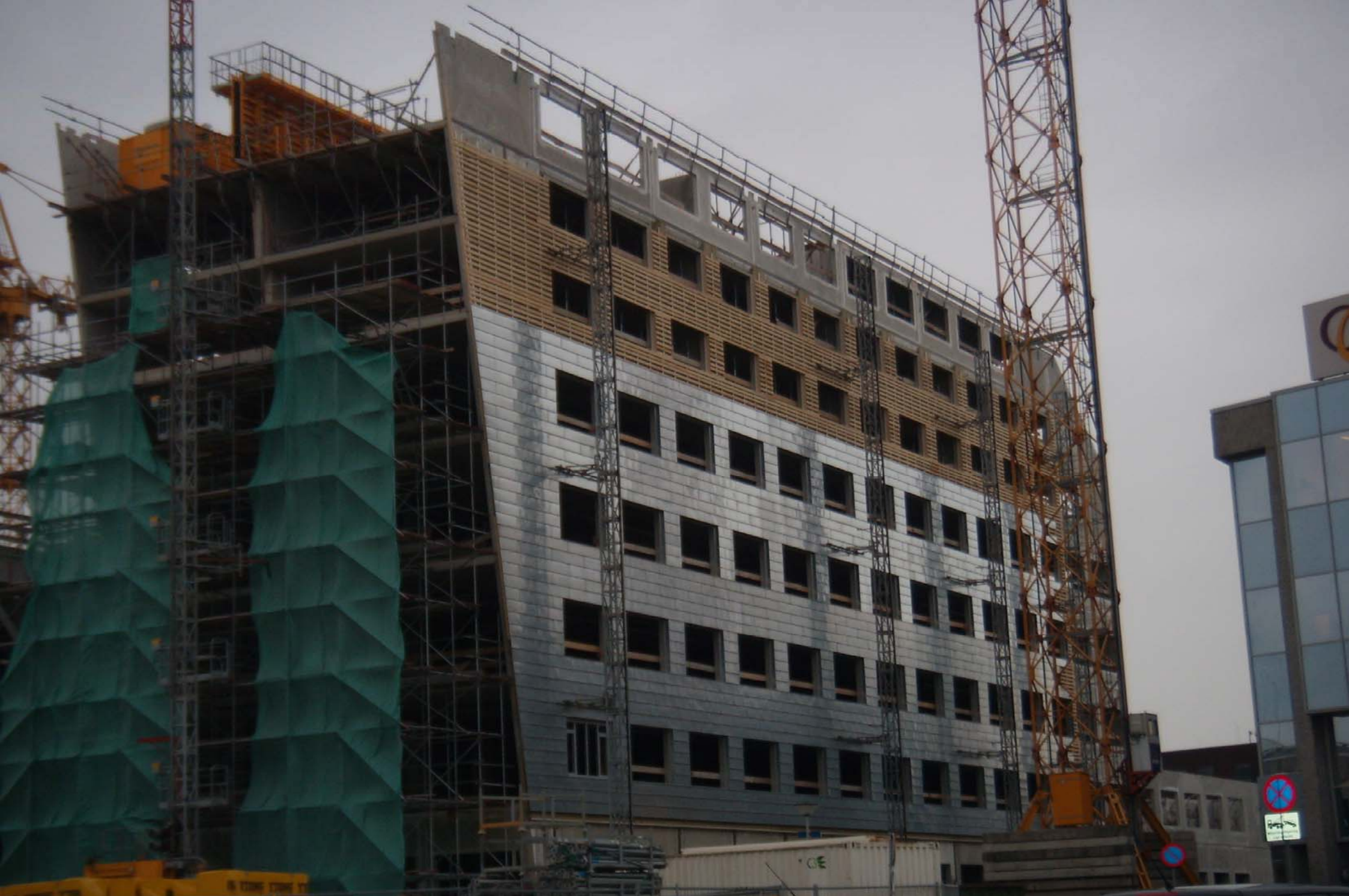
Office Building Turfship, Breda / Netherlands, Zinc, F1.10
